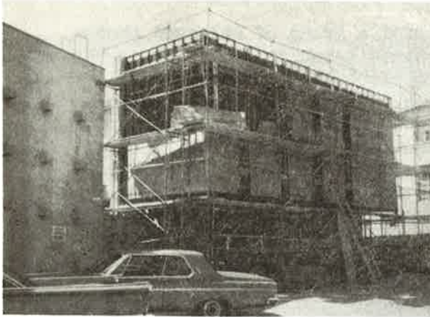
New construction on Los Feliz side of Headquarters.
