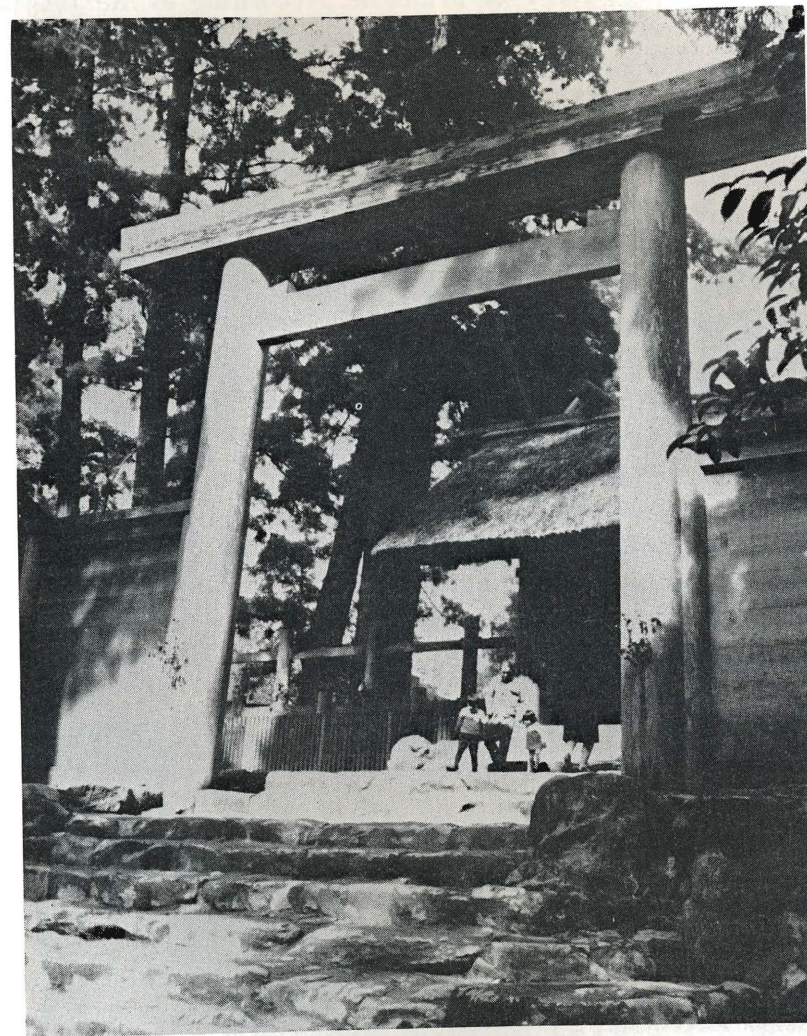
Torii at the Grand Shrines of Ise. The rustic nature of these structures is typical of ancient Japanese architecture.
