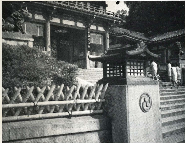
The Main Entrance to the Gion Shrine.
